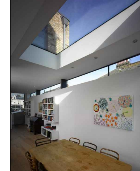
flat glass roof panel internal
