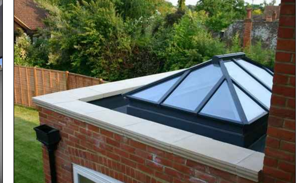
decorative coping stone on facing brickwork
